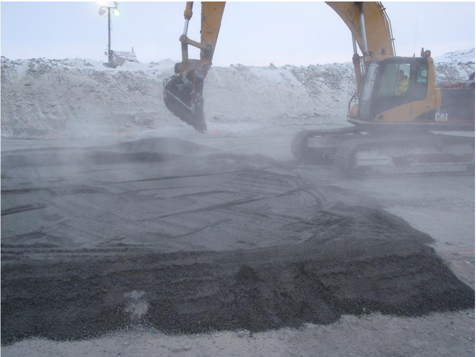
Photo 6: The first few lifts of FCM. Note the overbuild in the foreground to ensure design lines are met.
