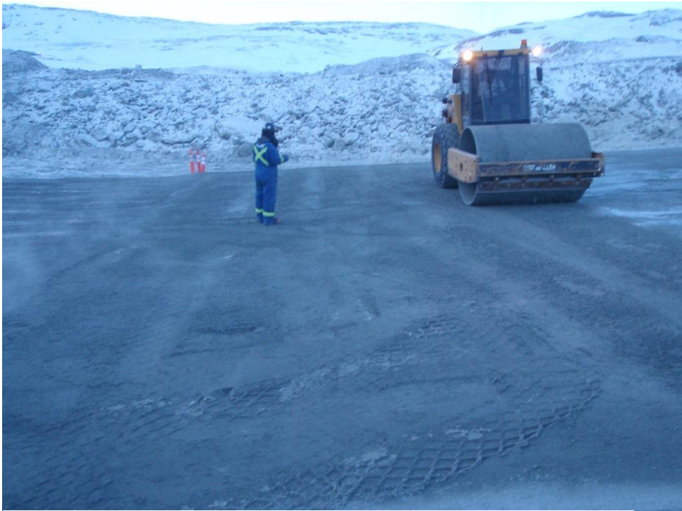
Photo 5: Area where saturation was low after initial compaction. Vibratory packer completed several extra passes to bring this area to passing specifications.
