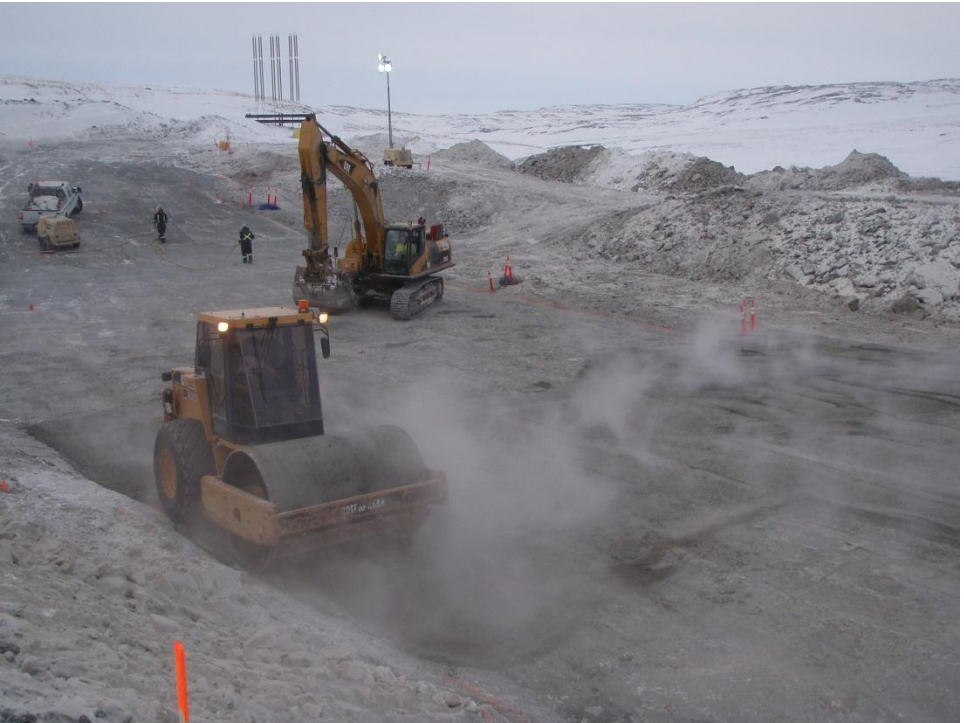
Photo 7: Vibratory packer passing four times with static rolling, two times with the vibrator on.
