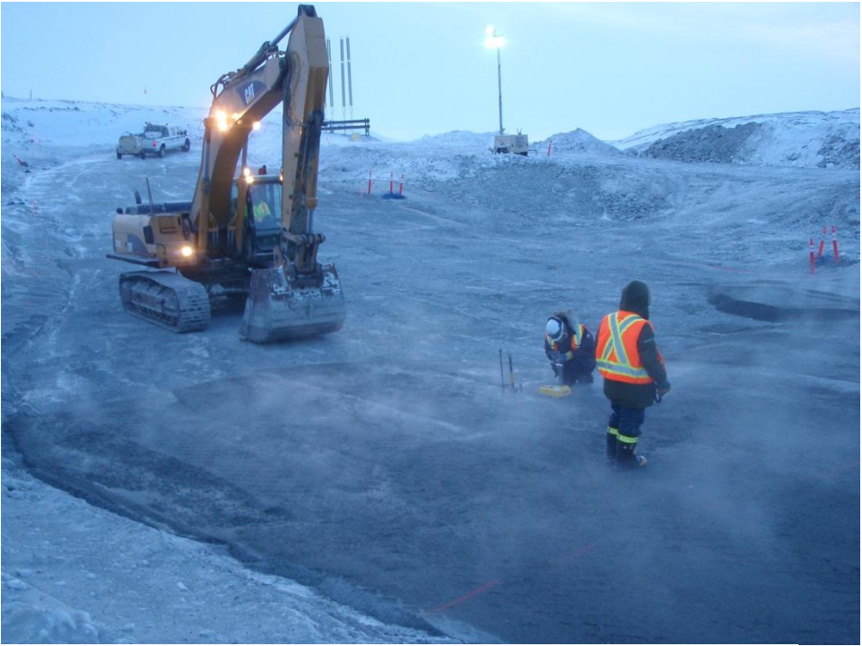
Photo 5: Midday placement of FCM. Nuclear density testing continued throughout placement.
